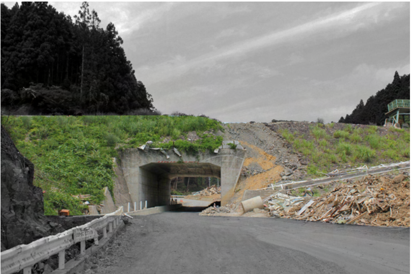
FRONT: Minor erosion happened, the gravel surface is slightly washed out.
