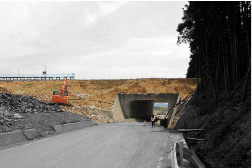
BACK: Serious erosion happened, the embankment surface is totally washed out, the soil infill is exposed.
