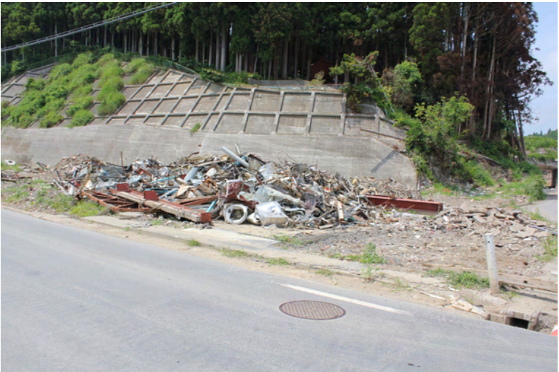
Concrete Retaining : Provides protection to prevent slopes from erosion , but its low wall porosity requires intensive drainage for rain
