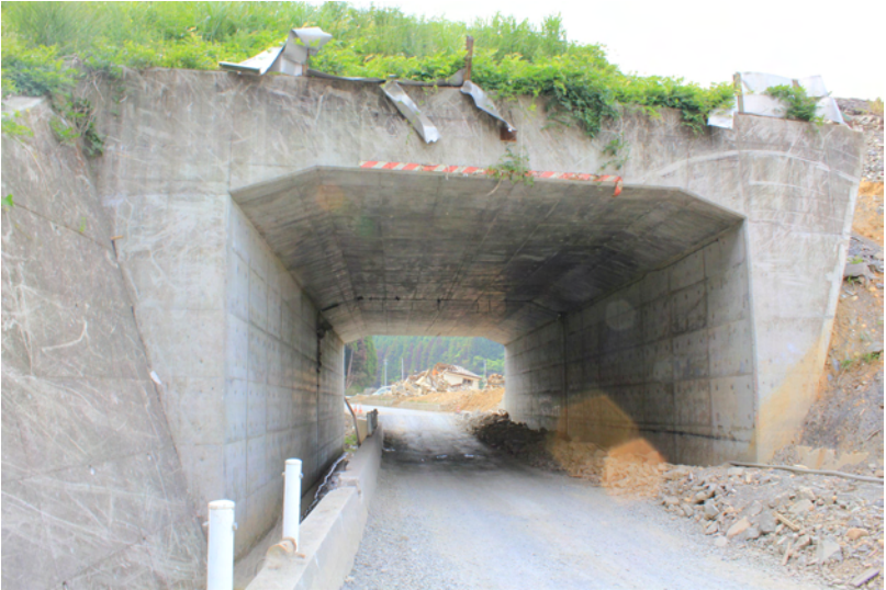
JR underpass: Becomes a by-pass for water when tsuinami came. It created a severe flush with high water velocity.
